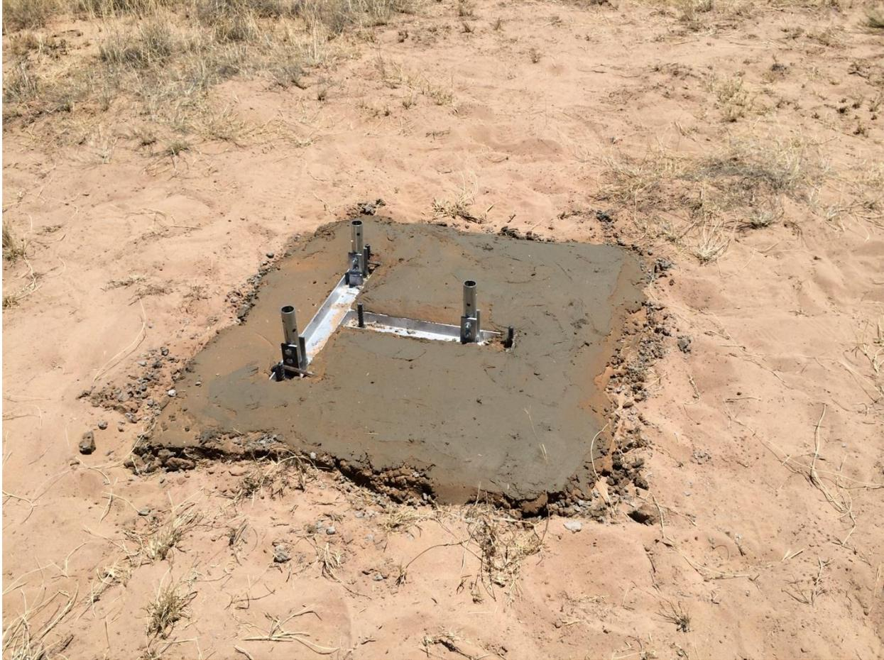
a. Parts Needed: Tower Base Plate, Base Plate Stakes, Rebar loops, Wood and Wire for Jig, Level (x2). Align Base plate in hole so that it faces South
